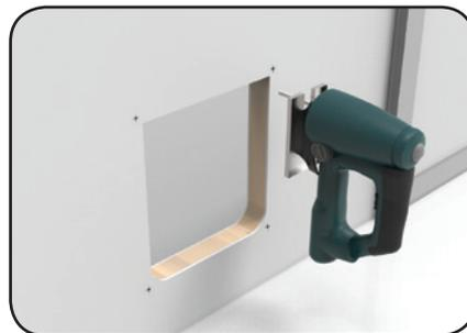
5. Using a reciprocating jigsaw, cut along marked lines.
