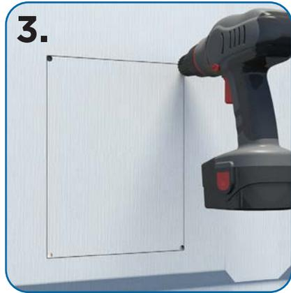
3. Drill a hole in each of the 4 inside corners with a minimum of 10mm drill bit.
